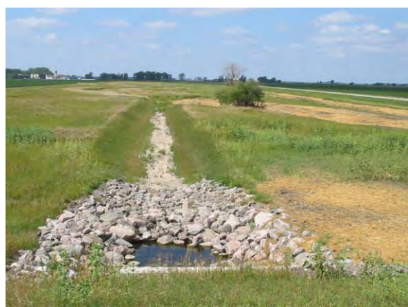
Principal Outlet structure looking west
