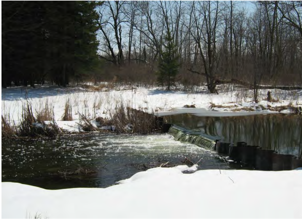
Stoplog sheet pile dam
