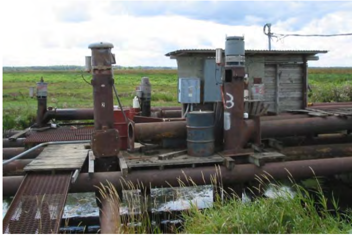
Typical pumping station
