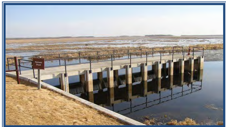
Stoplog Outlet Structure
