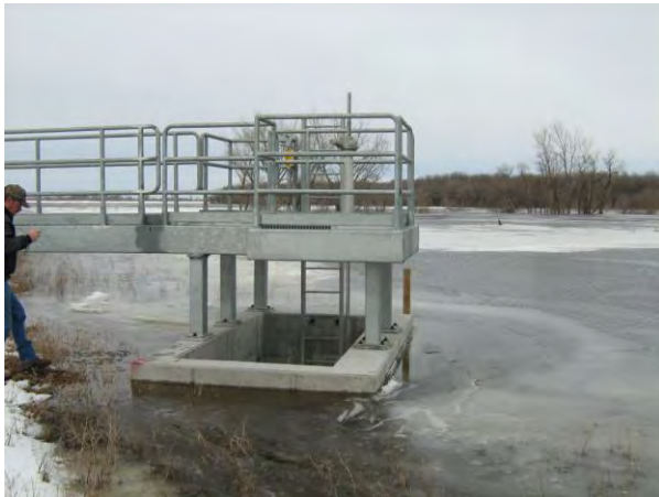
Full pool - frozen structure
