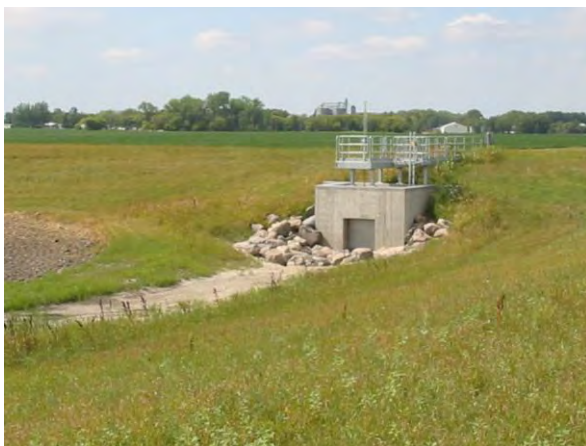
Principal Outlet Structure
