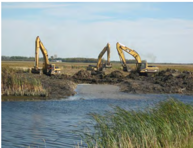
East pool excavation
