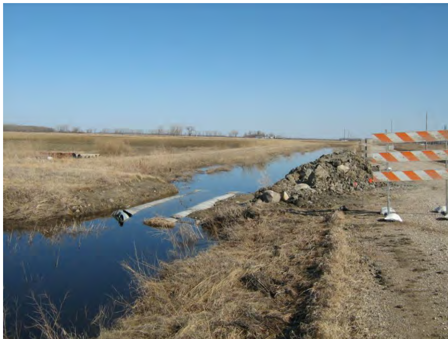
Parnell Impoundment culvert & field entrance damage
