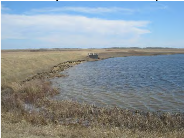
North levee wall repair needed
