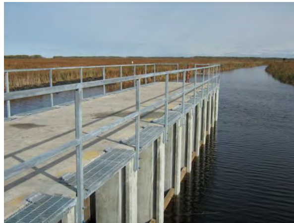
New safety grates and handrails installed
