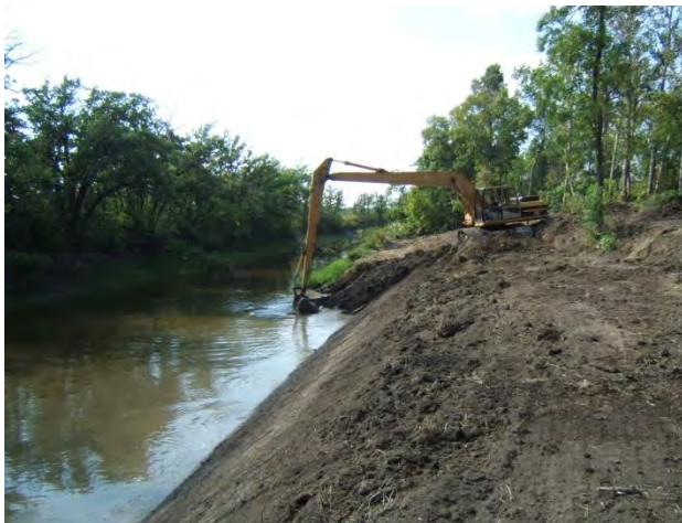
Removing a large silt bar from the channel.
