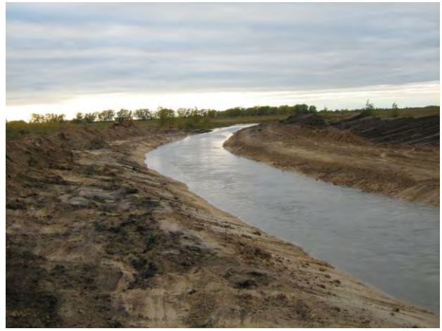
West pool interior channel
