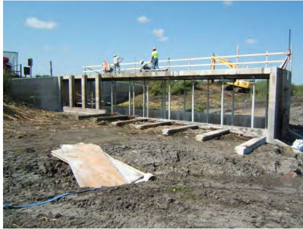
Concrete column and stoplog channel repair
