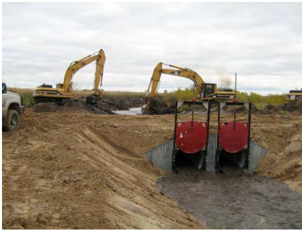
Installation of 2-48" gates culverts
