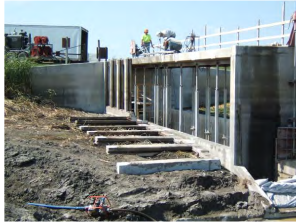
Concrete column and stoplog channel repair
