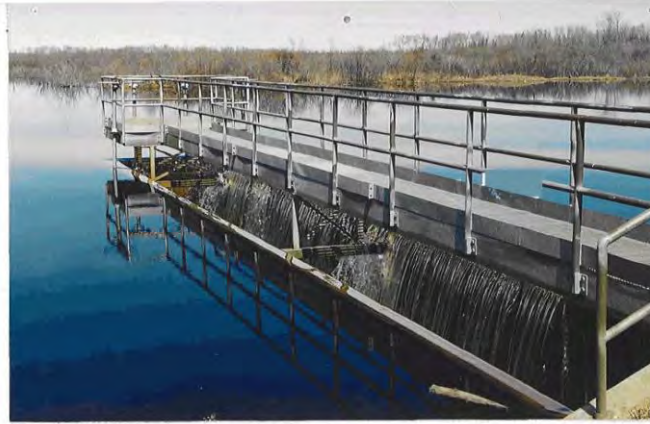
South Pool - Gated Principal Outlet Structure
