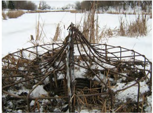
Control Structure needing repair
