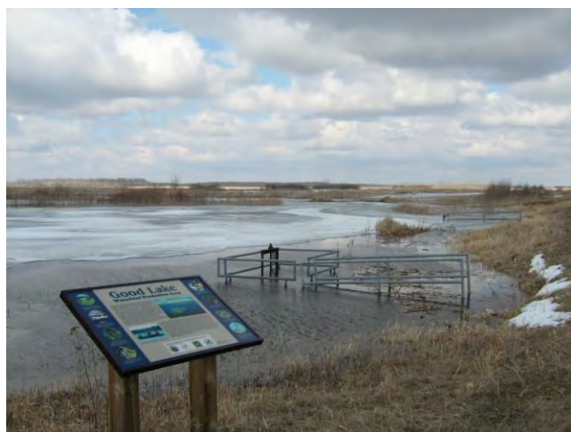
Gated Principal Outlet Structure
