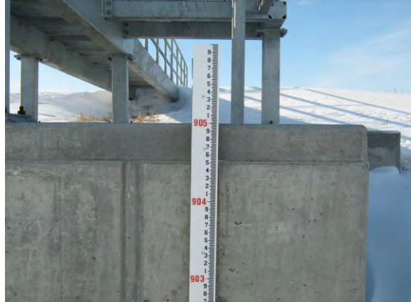
Typical staff gage at structure
