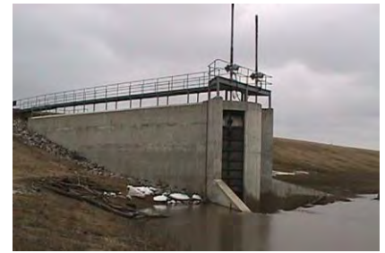
Principal outlet structure hydraulic gate operation
