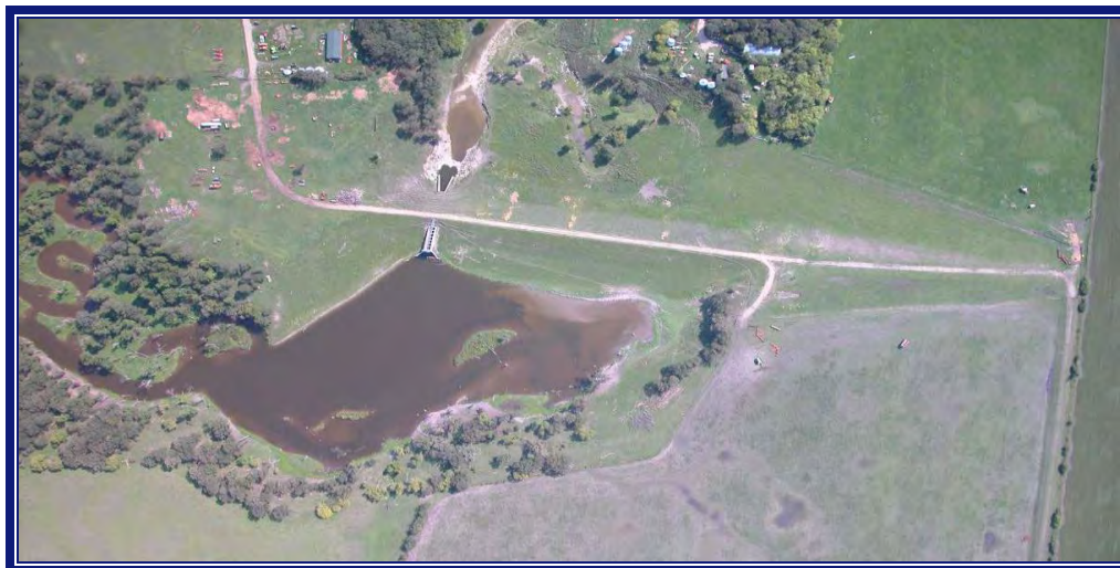
Aerial view of Schirrick Dam looking south
