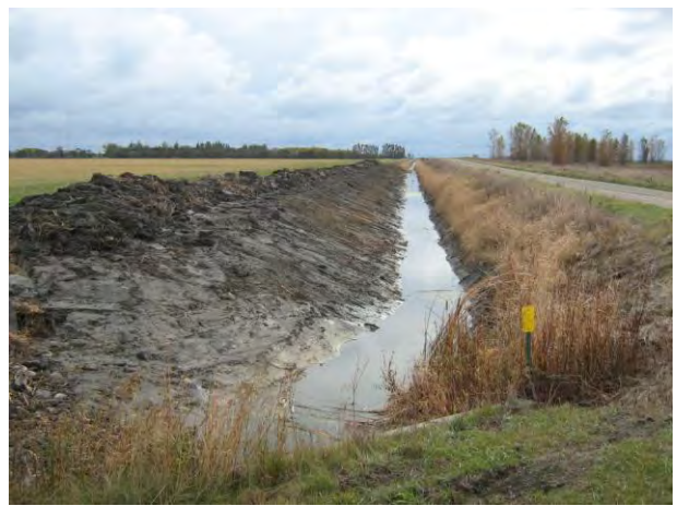
Judicial Ditch 60 cleaning
