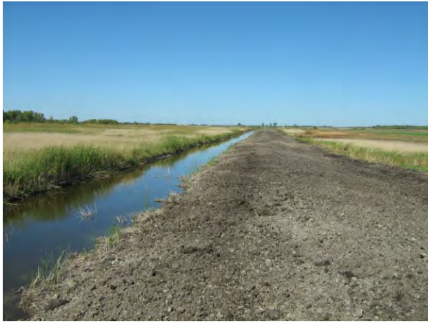
East pool interior ditch to enhance flow conveyance
