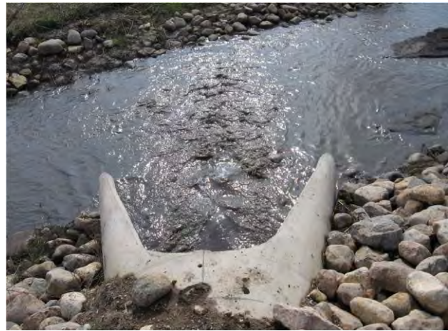
East Grand Forks Lift Station Outlet
