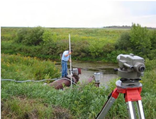
Surveying water lift from river to pump
