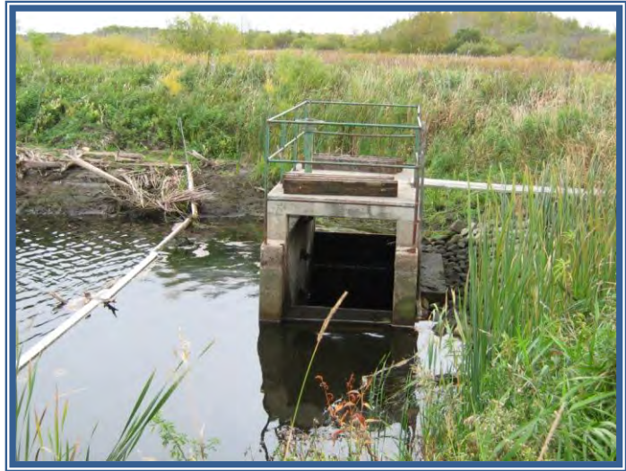
Outlet Structure/Pool Drawdown
