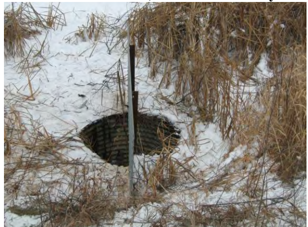
Install trash guard
