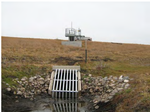
Critter guard installed on inlet end of structure
