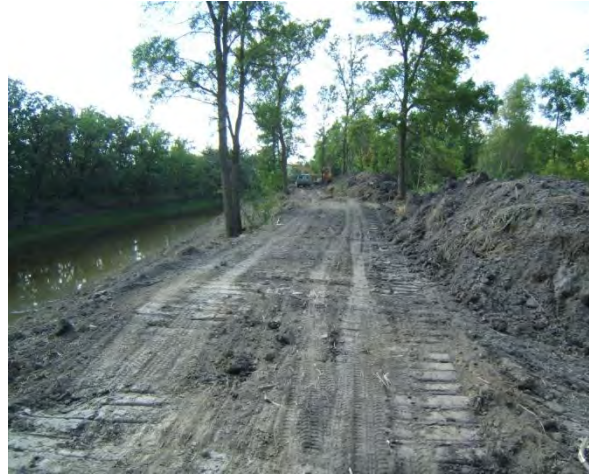
Ditch slope cut with spoil to be leveled.
