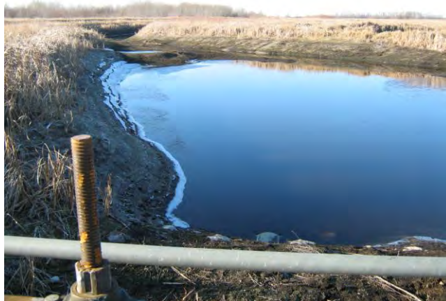
Gate open, damaged stem and pool drained due to vandalism
