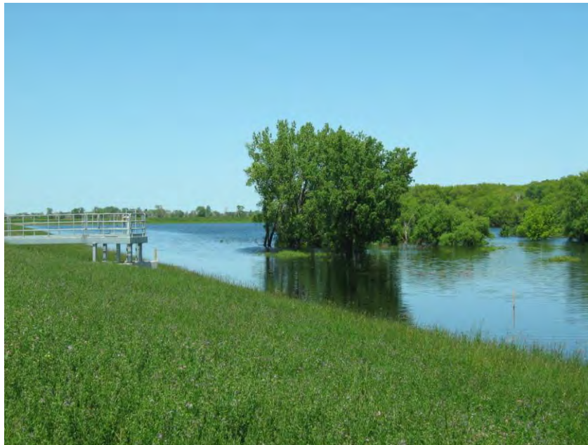
Principal Outlet Structure
