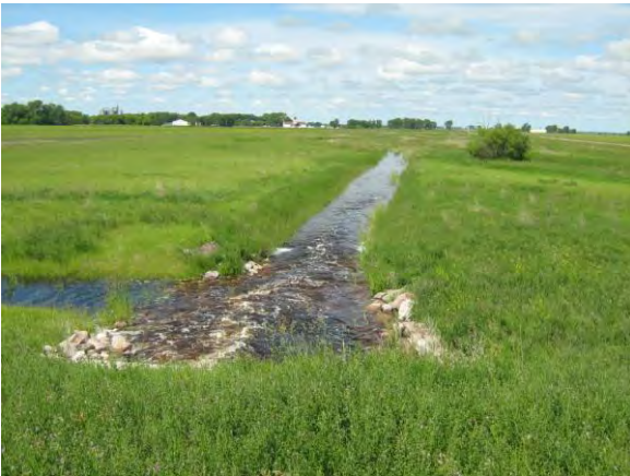
Controlled outflow from the impoundment
