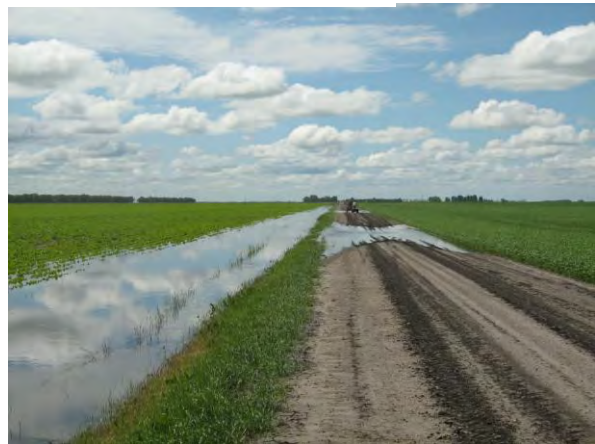
Flooded field/township road-Euclid Twp., Polk County
