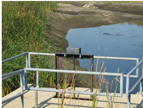
Screwgate locking device
