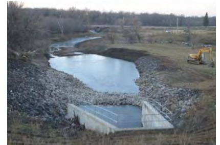
Looking downstream from outlet structure
