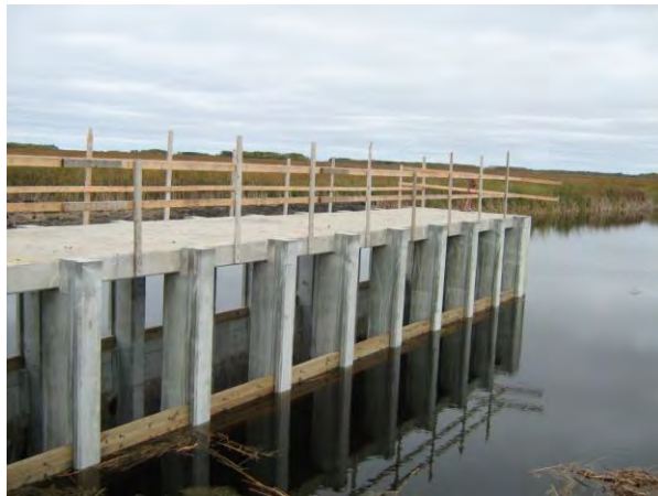
Column and stoplog repair completed
