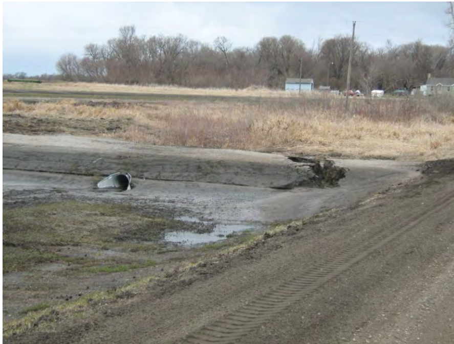
Brandt channel dike erosion
