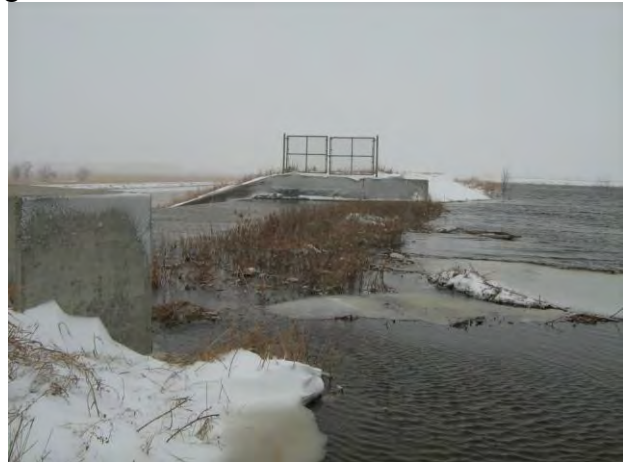
Concrete spillway water elevation 939.75
