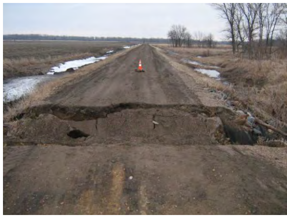
Culvert washout, Onstad Twp. Polk County
