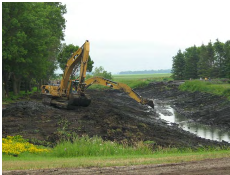
Typical Ditch Excavation
