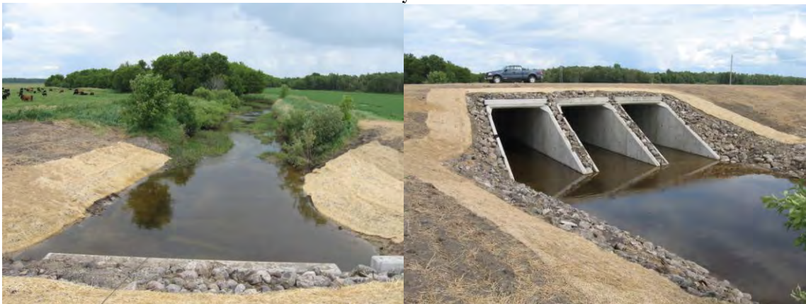
Mud River at Hwy 89 after construction
