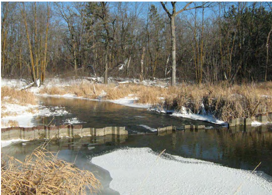
Stoplog sheet pile dam
