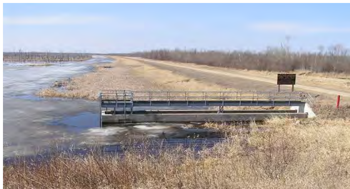
North Pool - Gated Principal Outlet Structure
